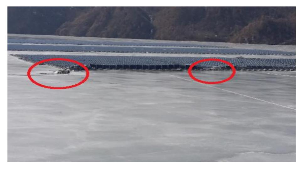
Ochang Reservoir Solar module damaged caused by ice pressure
