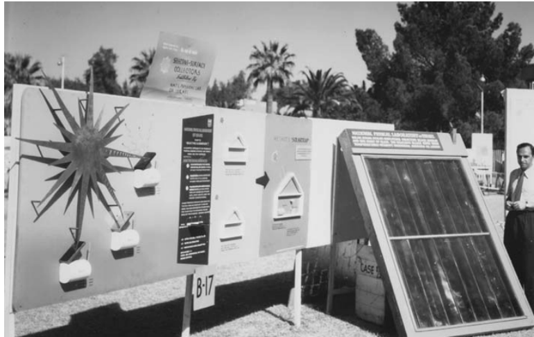
Figure 3: Harry Tabor with a flat-plate selective-surface steam generator at the “Sun at Work” exhibition at Phoenix in 1955
