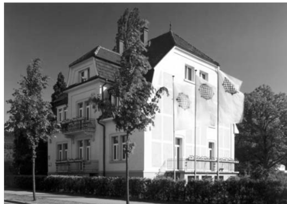
Figure 49: Villa Tannheim in 2000. Transparent thermal insulation is just visible on the wall behind the ISES Flags
