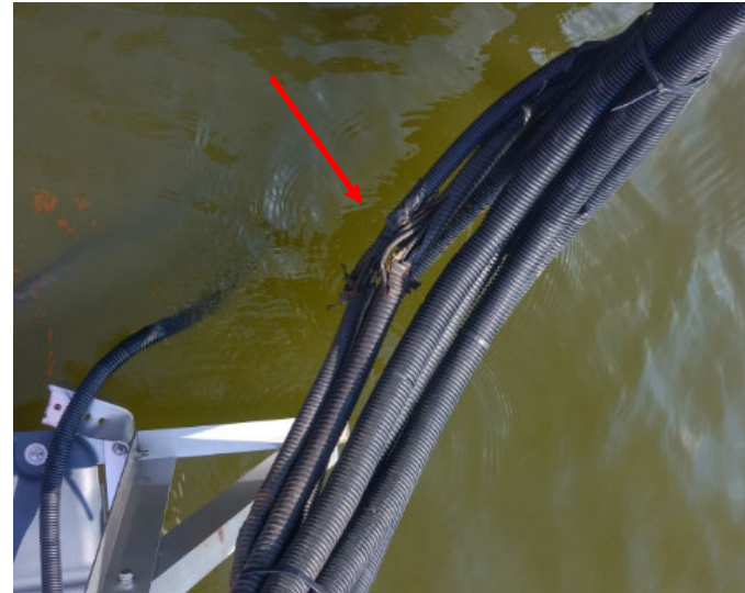
Damaged sheath
