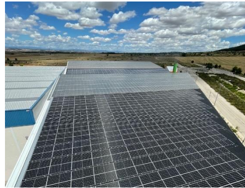
3.5 MW solar air PVT system drying animal food by Solarwall Spain
