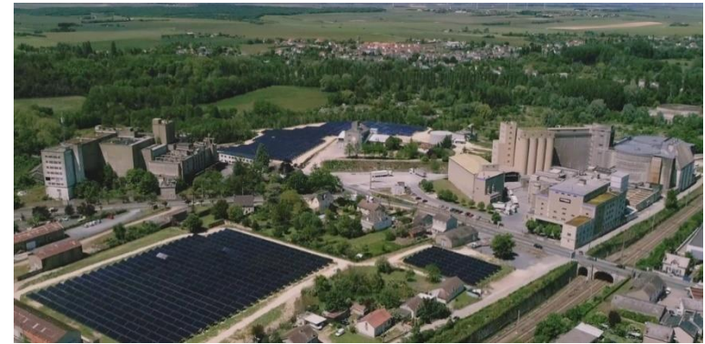
10 MW for air drying for malting plant in France by NewHeat/Kyotherm (ESCO)
