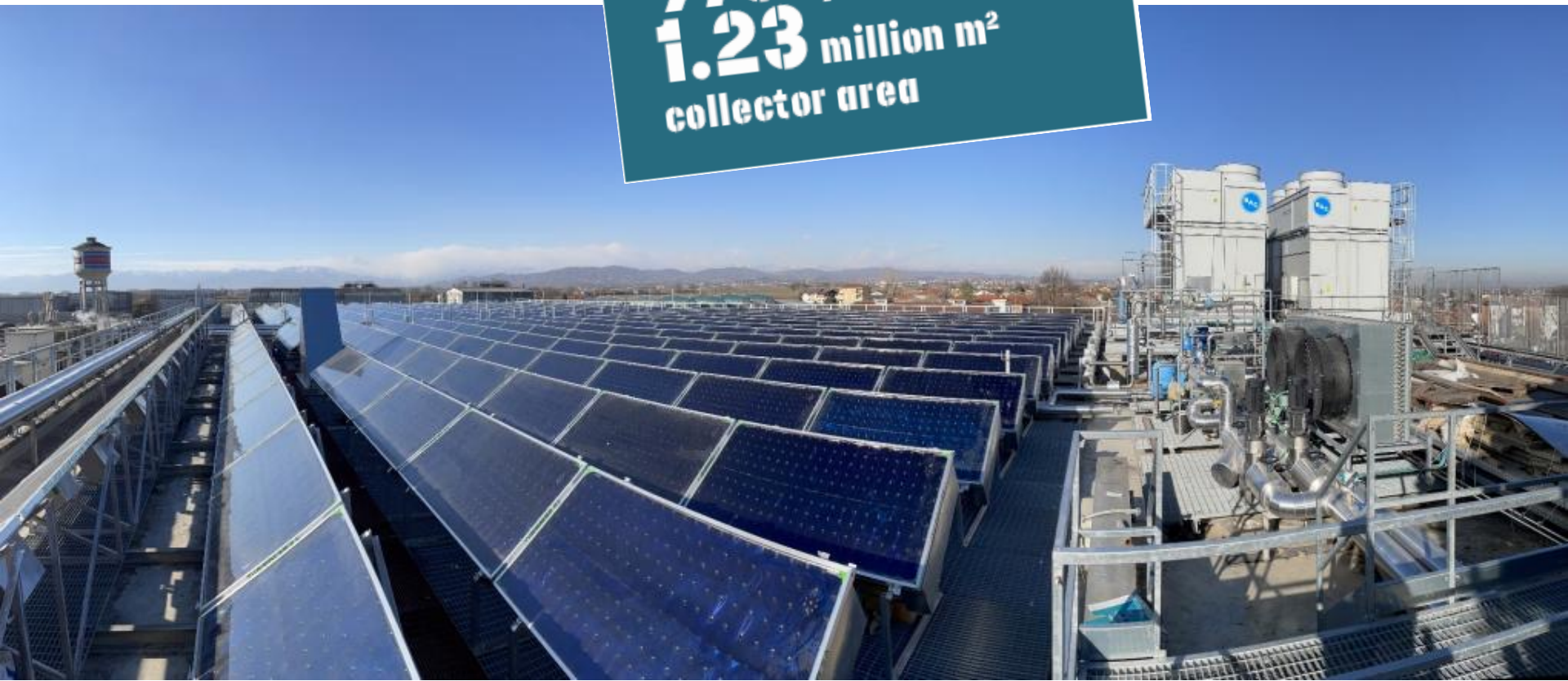
Solar process heat system for Martini & Rossi with a capacity of 0.42 MW th and equipped with high-vacuum flat plate collectors in Turin, Italy Photo: TVP Solar, Switzerland
