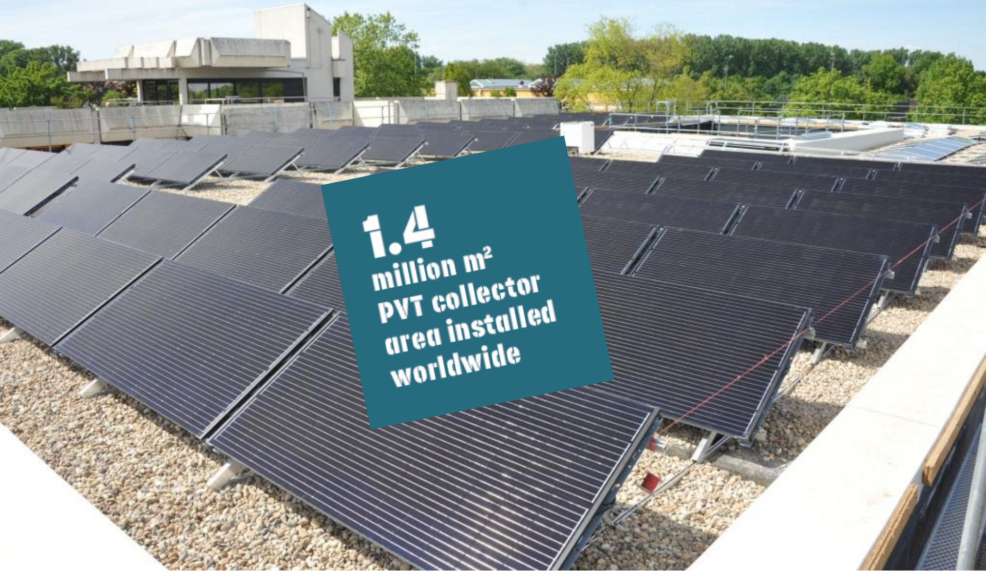
200 m 2 PVT-collector field for a new office/council building in Offenbach, Germany / Photo: Consolar, Germany
