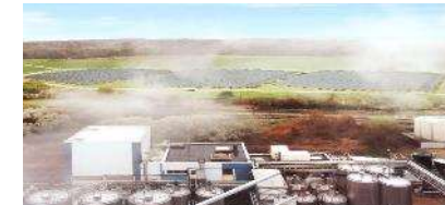
Spray drying site for dairy ingredients Grand Est region Peak power : 13,1 MWth Start of construction : Summer 2021
