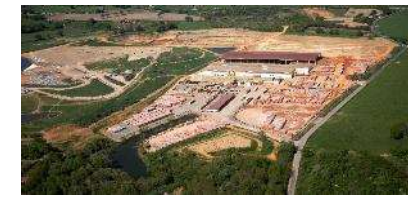
Terracotta brick production site (dryer and ovens) Auvergne Rhône Alpes region Peak power : 7,8 MWth Start of construction : Summer 2021
