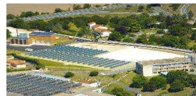
District heating – City of Pons (DALKIA) Pons, Charente-Maritime Peak power : 1,4 MWth Start of construction : Jun 2020
