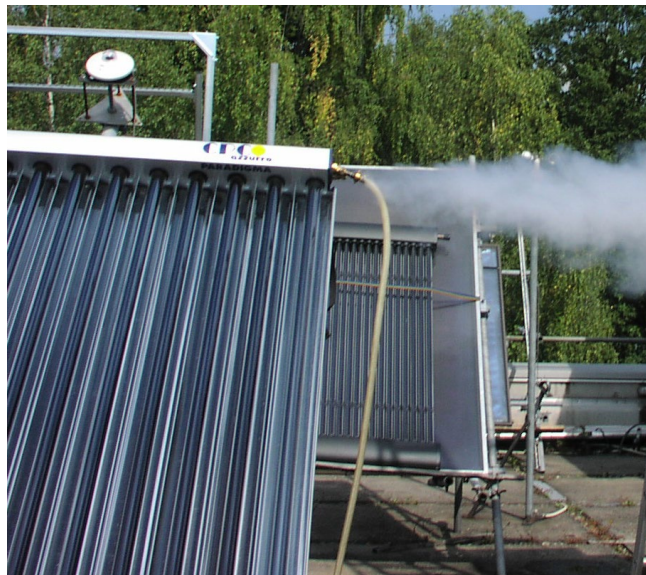
Flushing the hot collector with cold water
