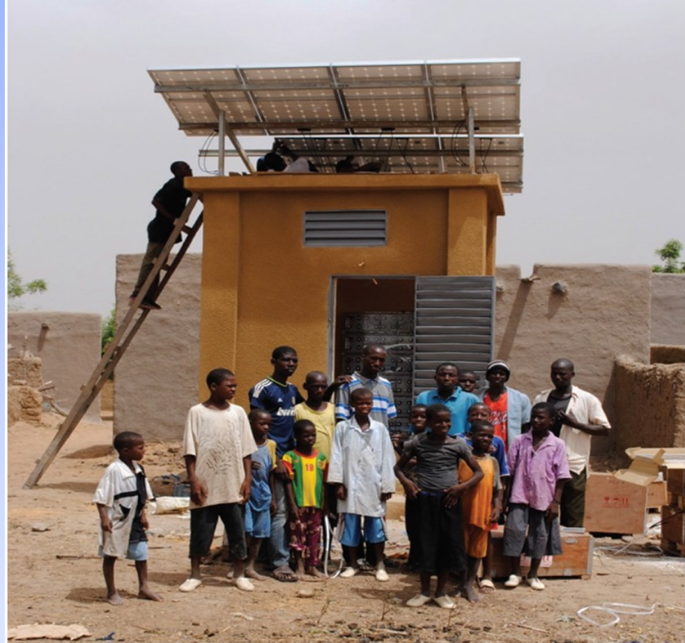
Figure 7.12 Shedsolar mini-grid installation during construction phase. Mali, 2011 (Source: Courtesy of V. Modi, Columbia University).
